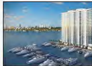
Marina Palms condo project taps Coastal Construction for second tower
